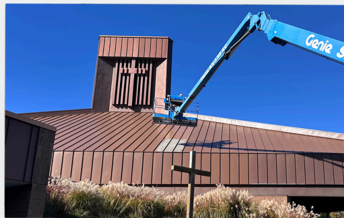
The roof being painted in the fall of 2025. Look at the difference!
